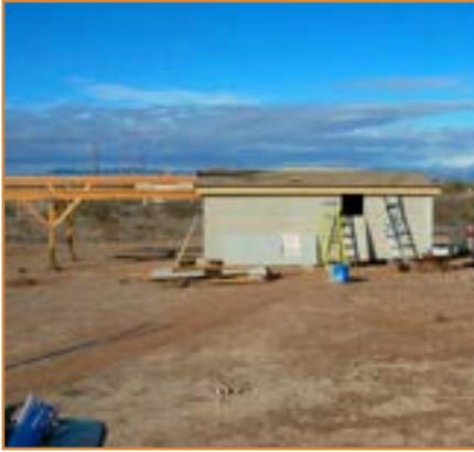
Two features which I believe are not common: 1) a fold down wall which interlocks with the roof rafters when the roof closes, and 2) a ramp to facilitate access by my Dobsonian on wheels as well as other wheeled machines.
