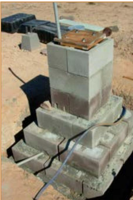
Rather than pour a foundation, Frank Pino suggested I simply use foundation blocks which I did. I wanted the floor to be as rigid as possible so I used 2x6 floor joists on 12 inch centers with  $\frac{3}{4}$  inch plywood over that for the floor.
