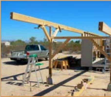
The roof is supported by 4-inch rollers, 5 on each wall/rail. The 2x4 rafters are on 12-inch centers for rigidity. The roof is standard construction of chip board, felt and composition shingles. It is heavy, but still manageable
